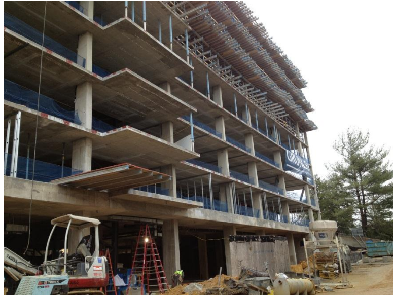
Figure 1: North Hall South Façade
